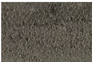
DRIVEWAY (NSW): COLOURED CONCRETE
